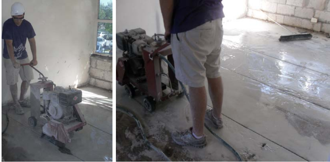
Figure A.32 – Saw-cutting of slab strips 1 and 2
